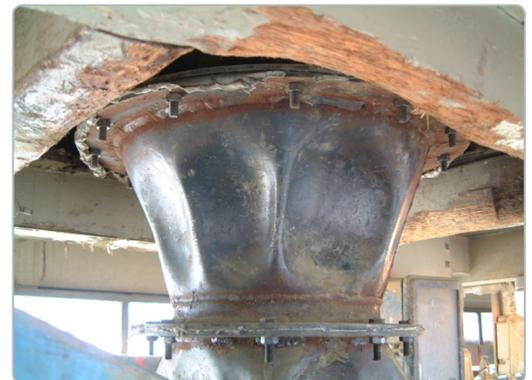
**Figure 2: Example of Hopper Suffering from Hammer Rash**
